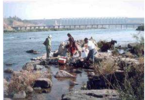
Plate 10: Bargi Dam Up stream
